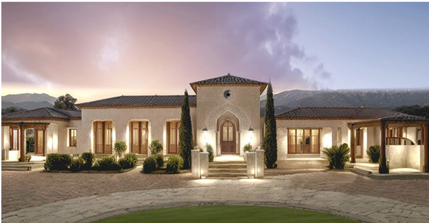
ALGODON ESTANCIA CURRENTLY UNDER CONSTRUCTION
